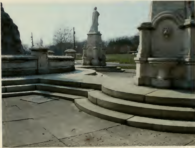
Figure 39: Granite stepped base (Photograph by author, March 2002)
